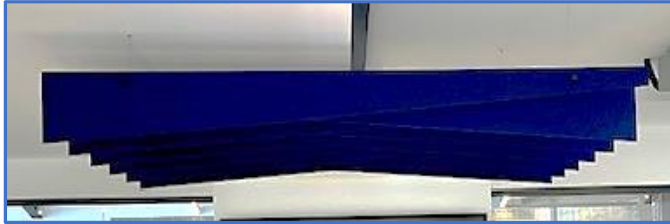
Acoustic Ceiling Baffles
